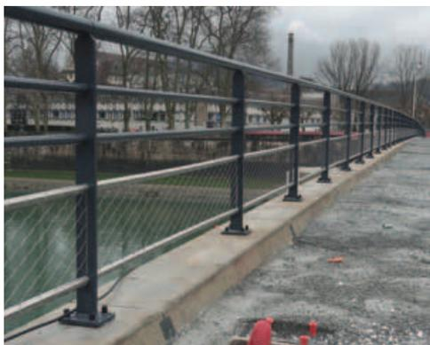
↑ POSE DU GARDE-CORPS SUR UN CÔTÉ DU PONT CANOT.
